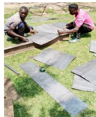
Metal fabrication (Fort Portal)
