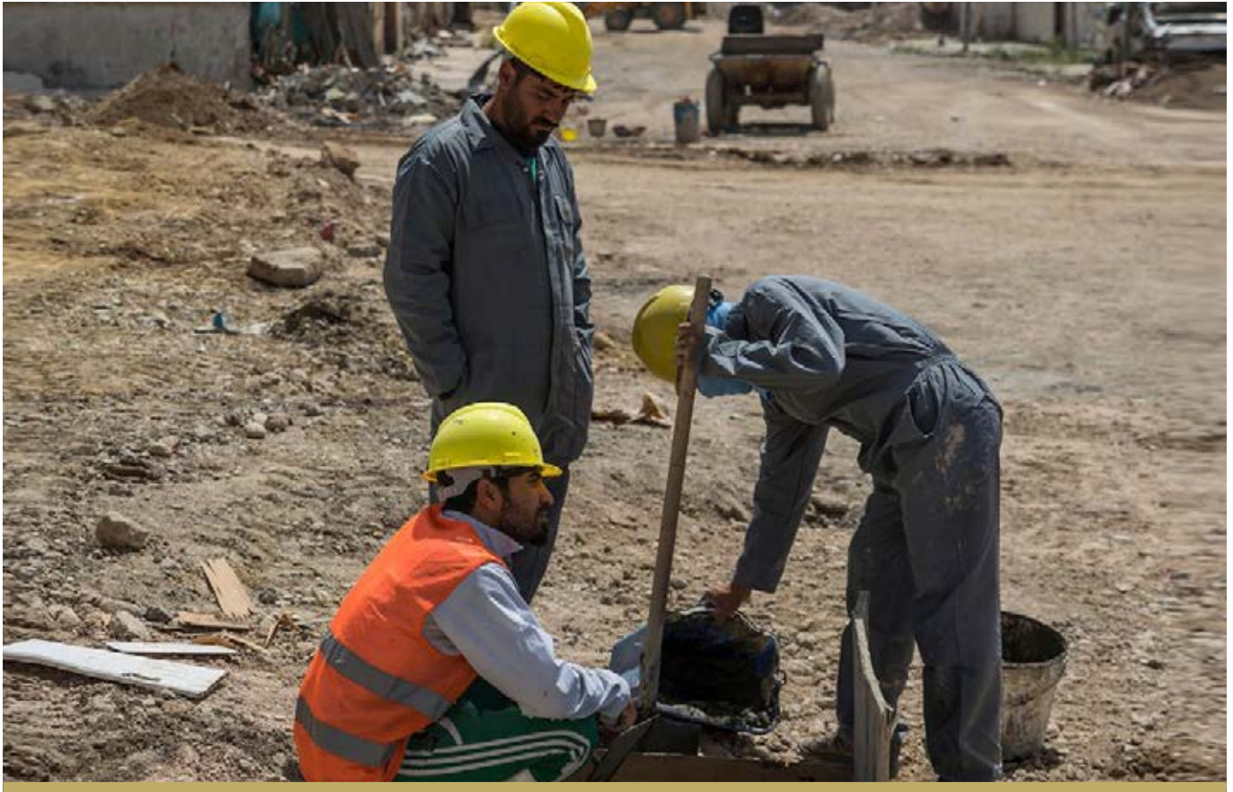
WORKERS REPAIR THE SEWERAGE SYSTEM AT THE WEST MOSUL HOSPITAL COMPLEX.
