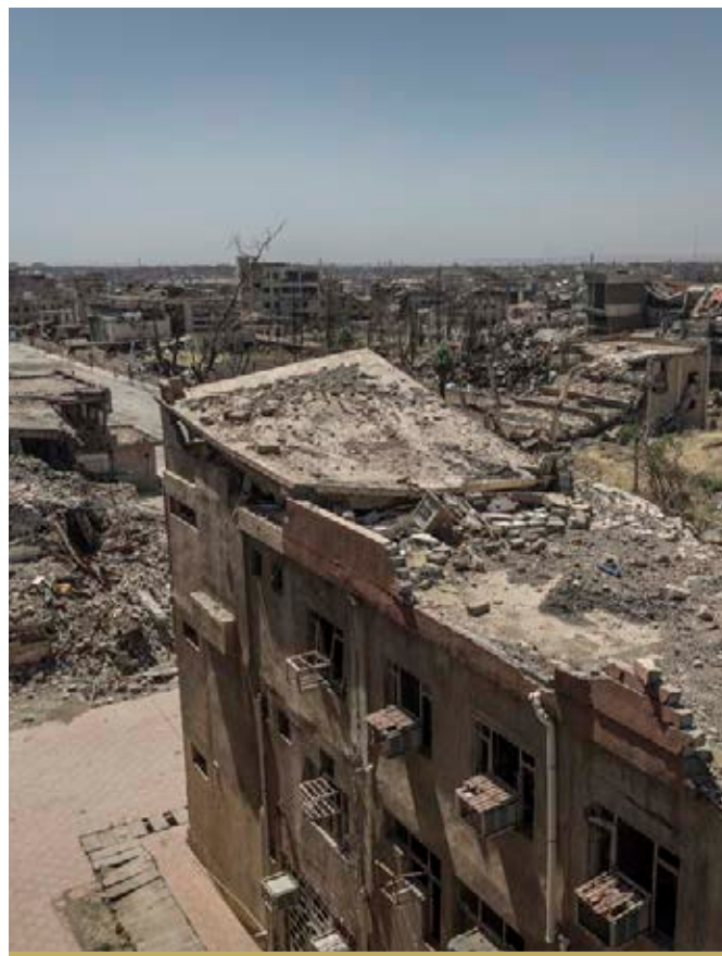
A VIEW OVER AL SHIFAA HOSPITAL COMPLEX. FFS COMPLETED THE ASSESSMENT FOR THE IBN SINAA HOSPITAL, THE ONCOLOGY HOSPITAL, THE AL BATOOOL MATERNITY AND OBSTETRICS HOSPITAL, THE BURNS AND PLASTIC SURGERY UNIT, FERTILITY CENTRE AND BLOOD BANK, ALL LOCATED INSIDE THE COMPLEX, IN 2018.
