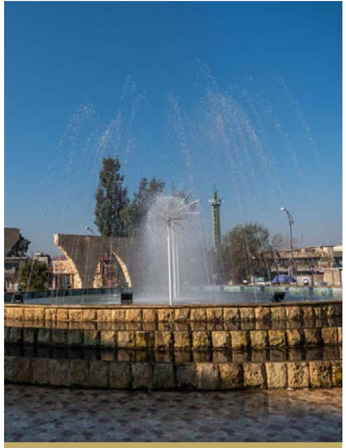
QUBBA ROUNDABOUT IN EAST MOSUL, WHICH HAS BEEN REHABILITATED IN 2018, INCLUDING REBUILDING THE ARCHES, FOUNTAIN, GARDEN PARK, LIGHTING, GROUNDS AND SEATING.
