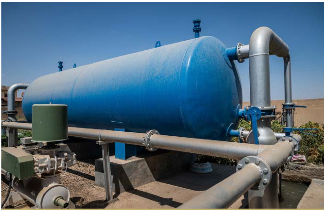
THE AL-FARIS WATER TREATMENT PLANT IN SHERGAT, COMPLETED DURING 2018.
