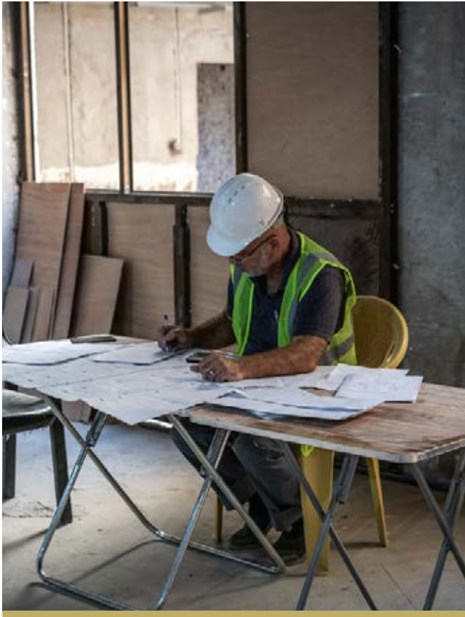
WORK ON THE MAIN BUILDING OF THE HOSPITAL WAS ONGOING, AND WAS 10% COMPLETE BY THE END OF THE YEAR.
