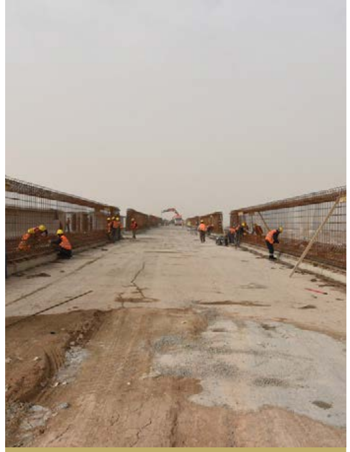
THE PALESTINE CONCRETE BRIDGE, AT 11% COMPLETION BY THE END OF 2018.
