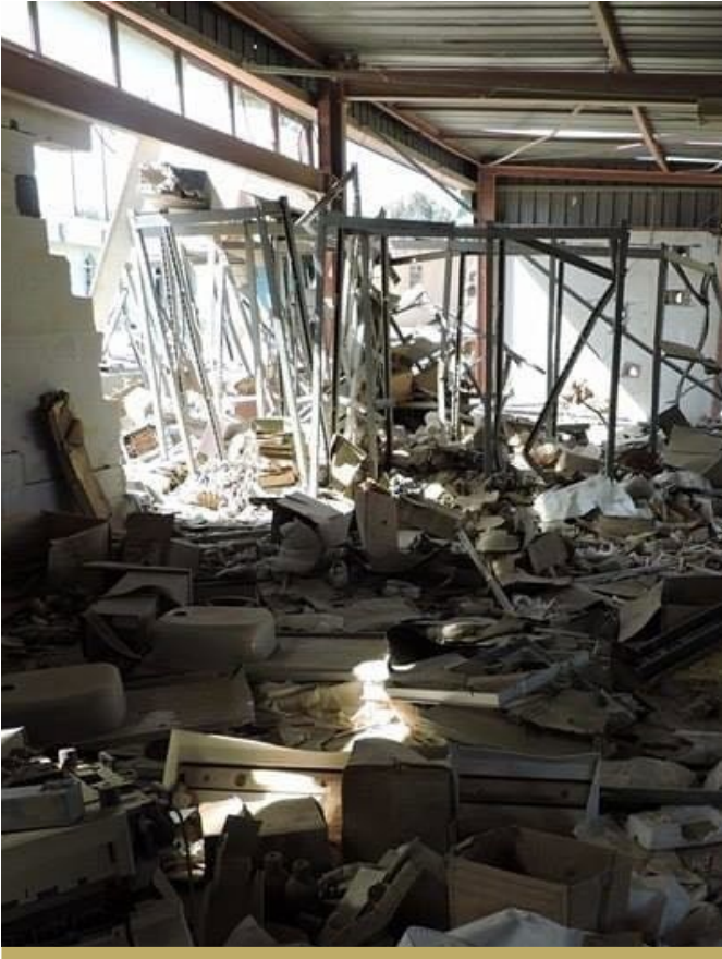
BEFORE: WORKSHOPS AT THE ANBAR TECHNICAL INSTITUTE, PRIOR TO THEIR REHABILITATION.
