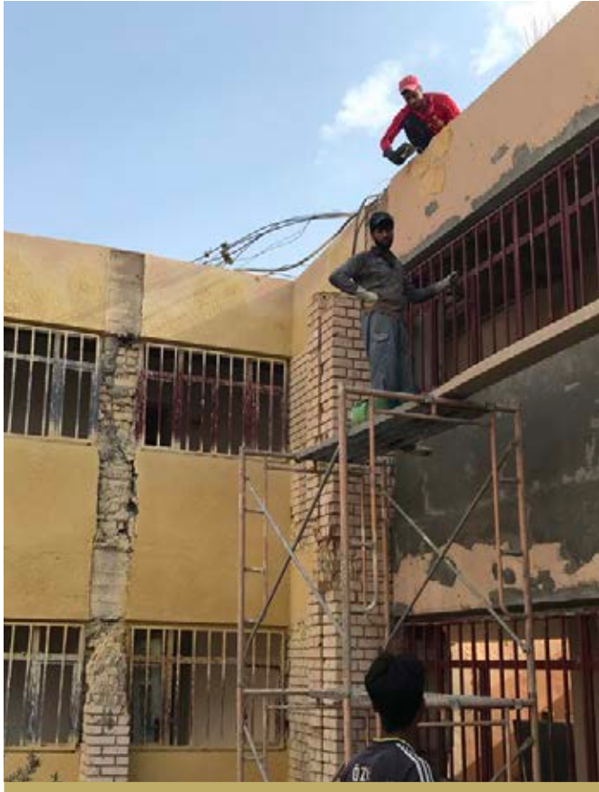
BEFORE: THE COLLEGE OF ADMINISTRATION AND ECONOMICS, WHILE WORK WAS ONGOING.
