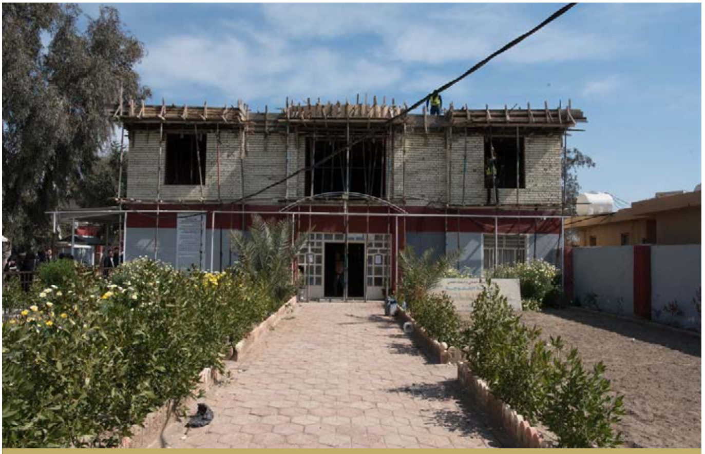
WORK IS ONGOING ON THE COLLEGE OF LAW AT FALLUJAH UNIVERSITY.
