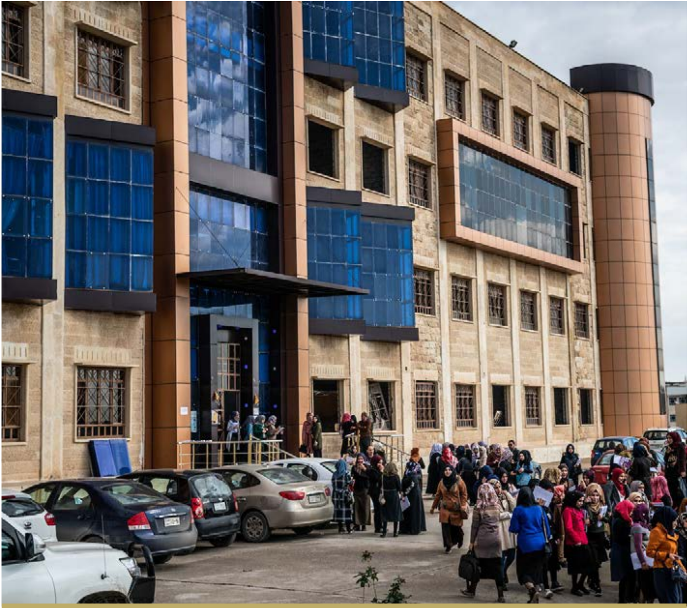
THE WOMEN'S EDUCATION FACULTY AT MOSUL UNIVERSITY, COMPLETED DURING 2018.
