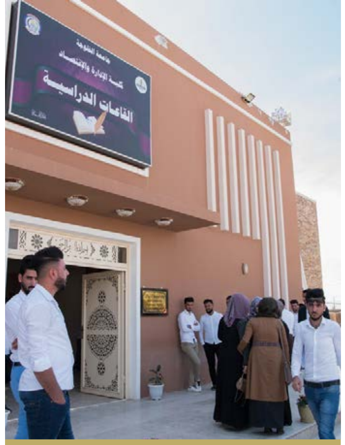
AFTER: OUTSIDE THE COLLEGE OF ADMINISTRATION AND ECONOMICS AT FALLUJAH UNIVERSITY, WHICH WAS REHABILITATED IN 2018.
