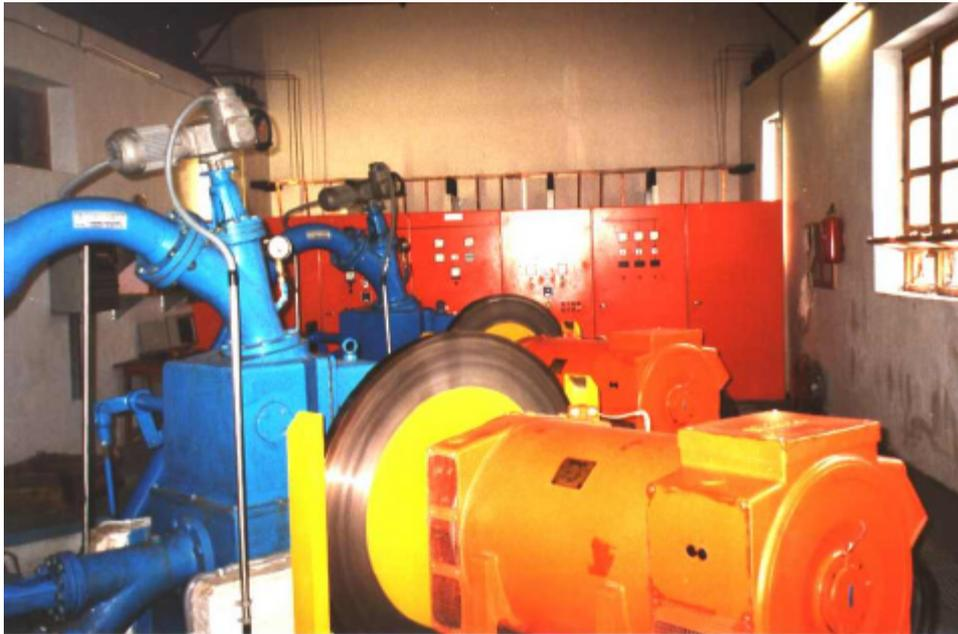
Figure 8: The two sets of double-jet Pelton turbines with synchronous generators, in the background the control and switch gear panels
