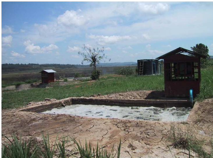
Effluent treatment plant at TALIU
